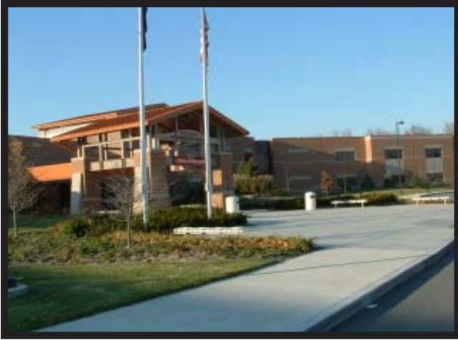
Educational Design Award Riverside Intermediate School Owner: Hamilton Southeastern Schools Mason: Ziolkowski Construction, Inc. Architect: Fanning Howey Manufacturer / Supplier: Edgewood Building Supply
